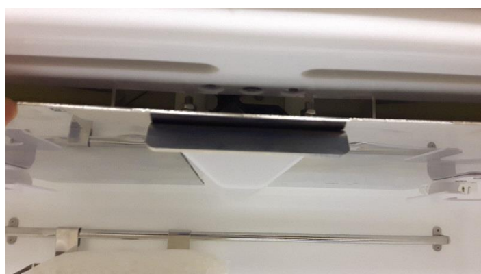
Figure 35: Ceiling Panel Handle and Grab Catch
